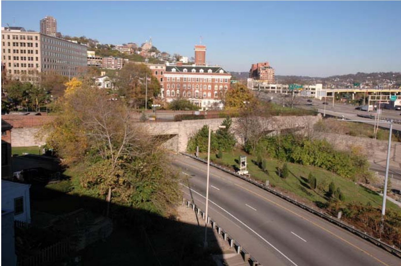
Park space over the highway tunnel
