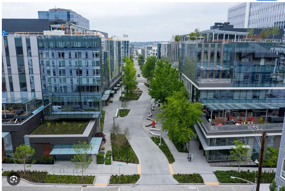
ArborBlocks S142040 04 C132040 01 N21 Construction Woonerf Street View |
