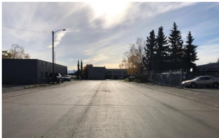
Figure 59. View of Hyder Street at 14th Ave in autumn (Image Credit: Allen Kemplen)
