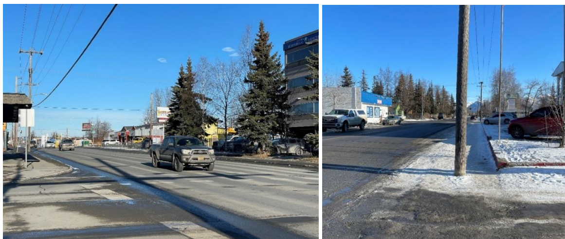
Figure 57. View of Gambell at the 13th Ave and a power line blocking a sidewalk in February 2025
