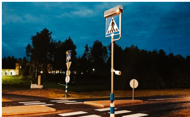
Figure 29. Warning lights with infrared sensors in Rauma, Finland (Image Credit: Rauma)
